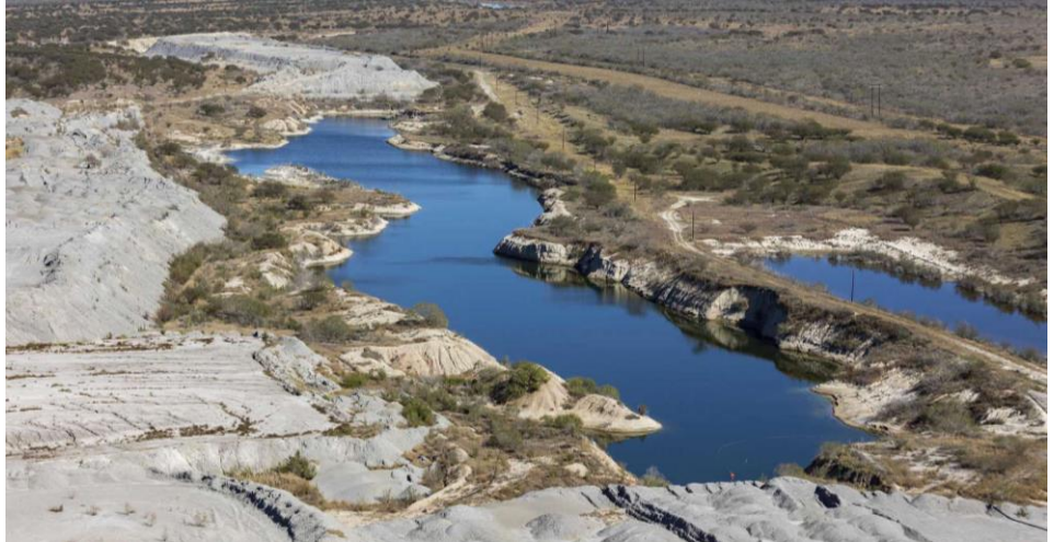
San Miguel Electric Cooperative's coal mine facility. Link
