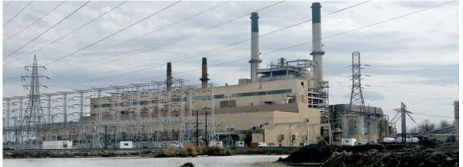
Ameren's Meramec Energy Center coal ash pond. Link
