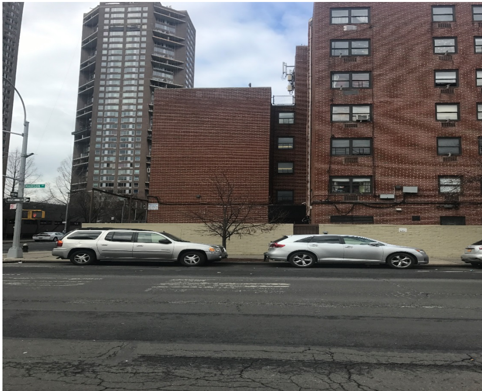
Photograph 5: View of adjacent property located to the southwest
