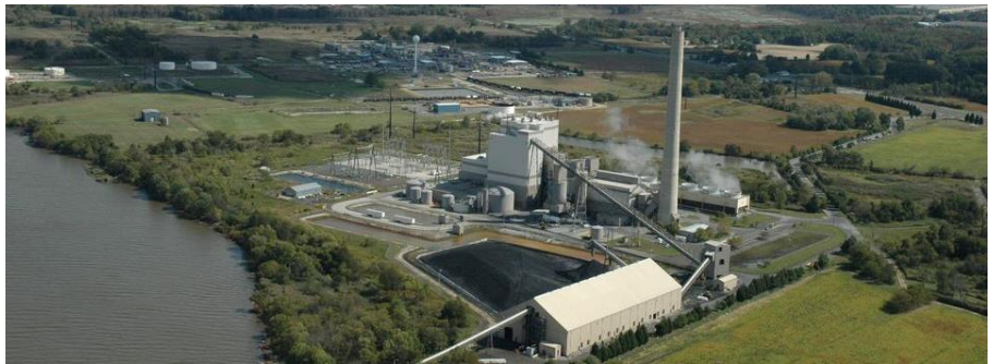
Logan Generating Station prior to controlled demolition. Link
