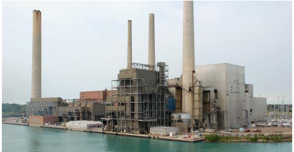
DTE Energy St. Claire Coal-fired Plant. Link
