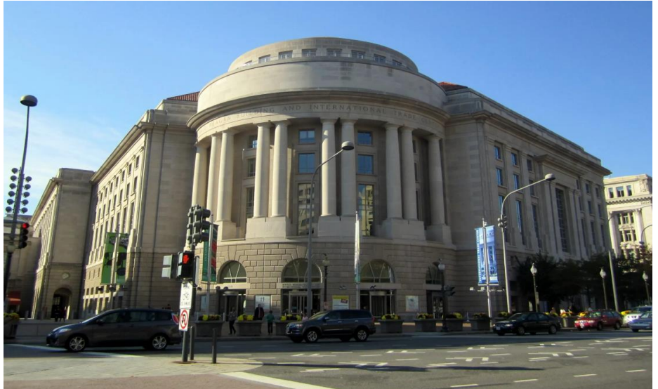
The Ronald Reagan Building, home to the EPA, was built with coal ash.
