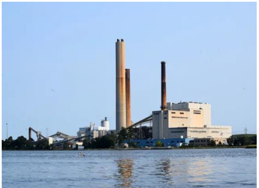
NRG Energy's Indian River Power Plant.
