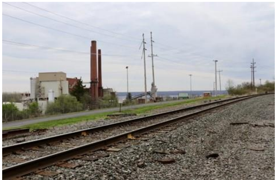
The Greenidge Generation bitcoin mining facility in Dresden, NY.
