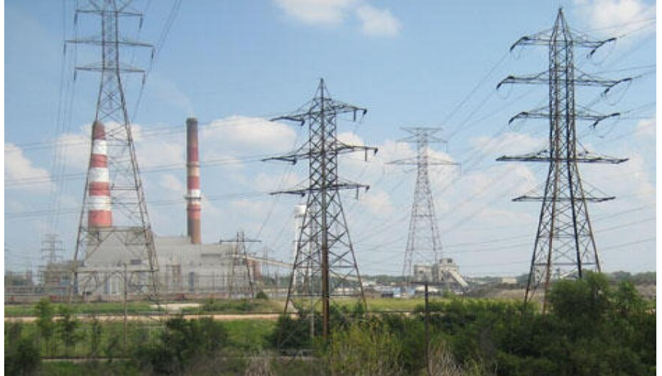
E.D. Edwards coal power plant near Bartonville, Illinois.
