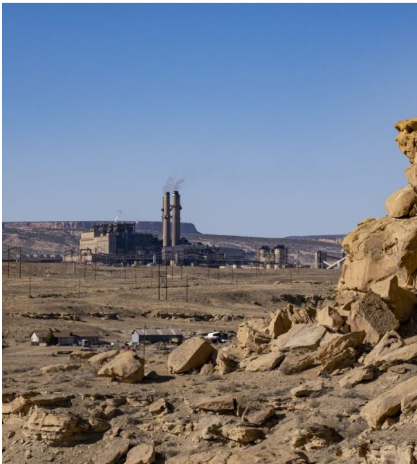
The coal-fired San Juan Generating Station in northwestern New Mexico. Link
