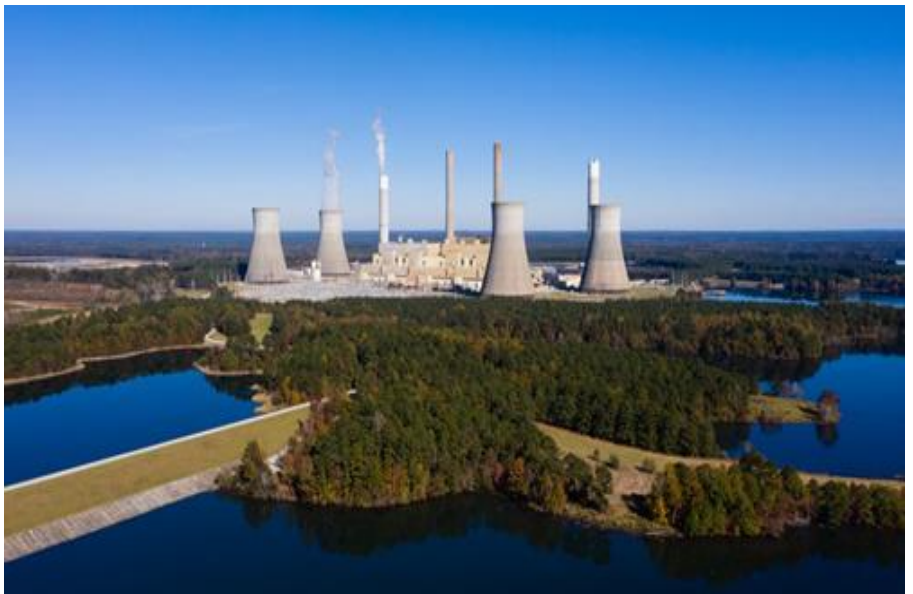
Plant Scherer, a Georgia power plant near Juliette, Georgia. Link
