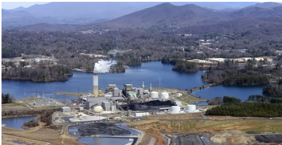
Duke Energy's Power Plant at Lake Julian
