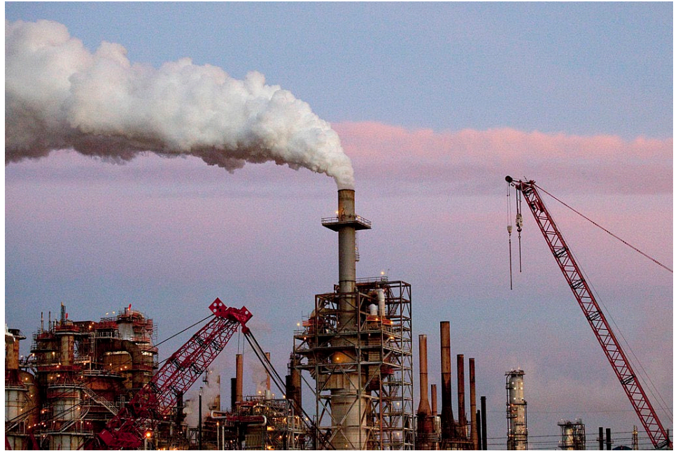
Petrochemical Refinery in Houston, Texas
