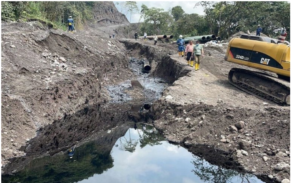
6,300 barrels of oil leaked into a natural reserve in Ecuador in a protected area of the Amazon
