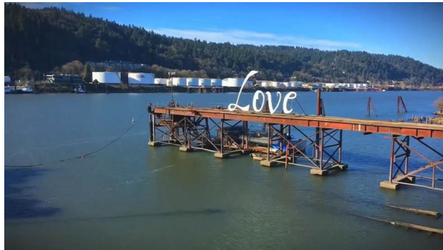
Critical Energy Infrastructure along the Willamette River, OR
