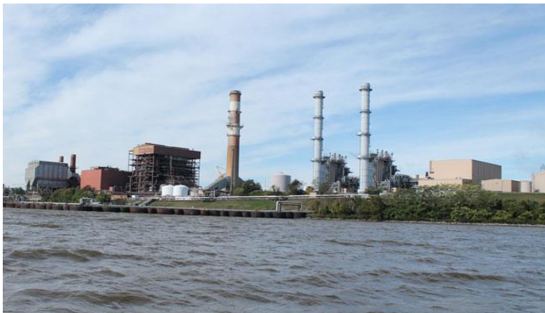
Dominion Energy's Possum Point Plant in Dumfries, VA
