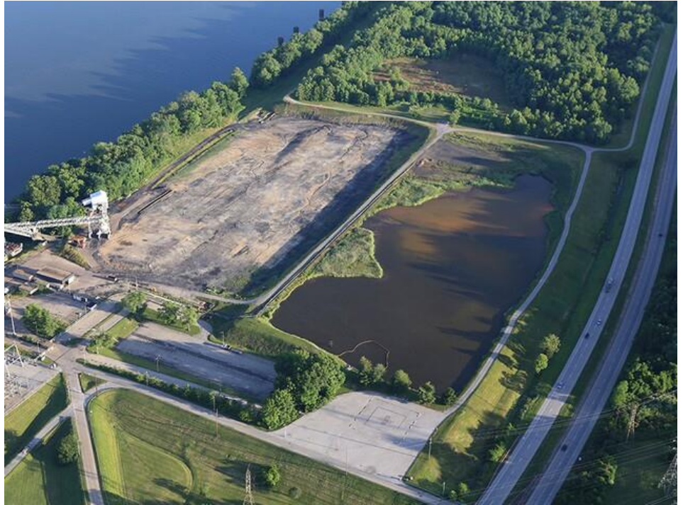
William C Beckjord Power Plant in Pierce Township, OH
