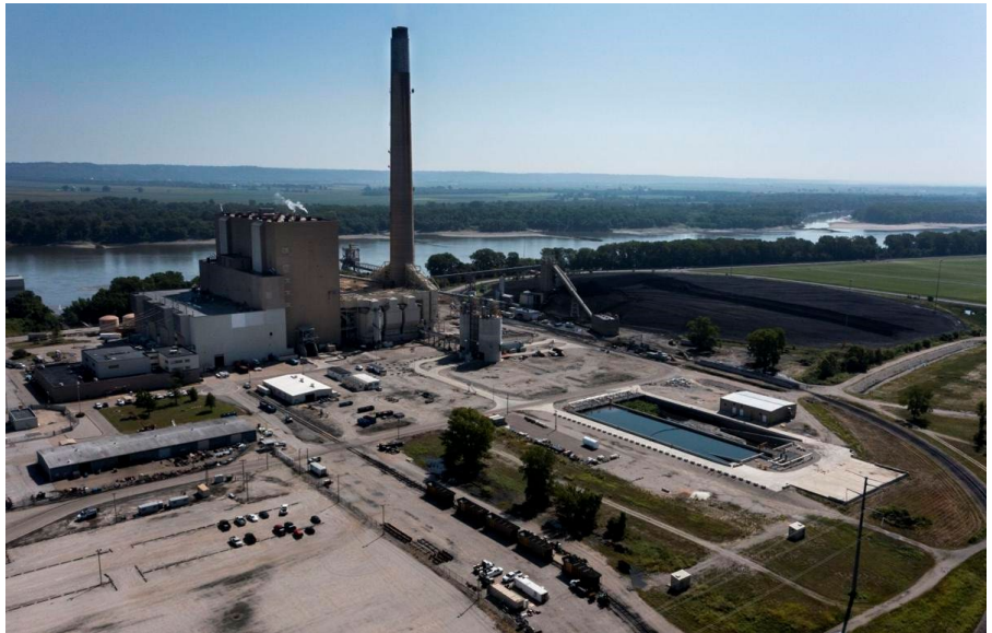
Ameren's Rush Island Power Plant
