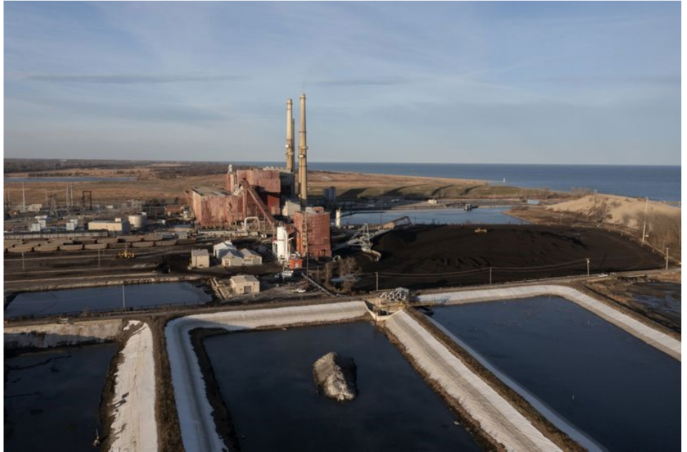
Waukegan Generation Station coal-fired plant in Waukegan, IL.
