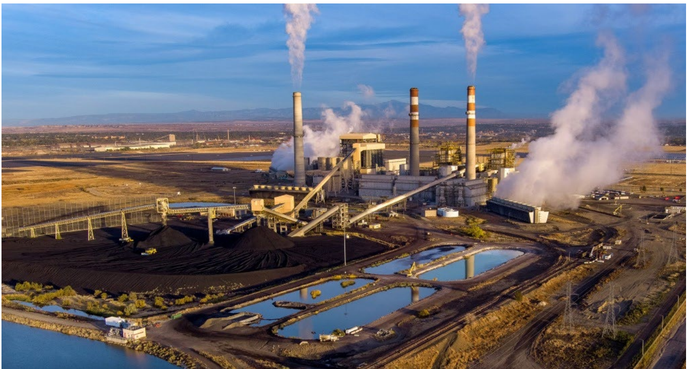
Comanche Generating Station in Pueblo, Colorado.
