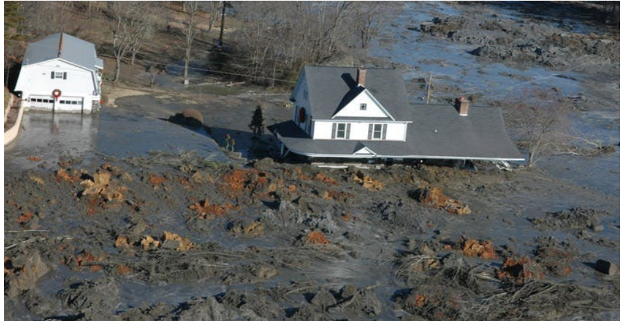
A 2008 photo of the Kingston coal ash spill.
