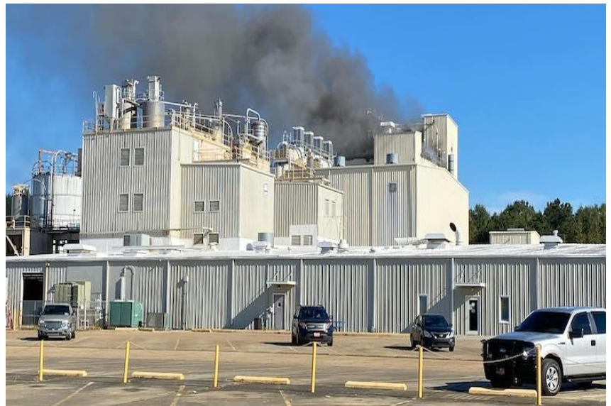
Westlake Chemical Plant in Gallman, Mississippi.
