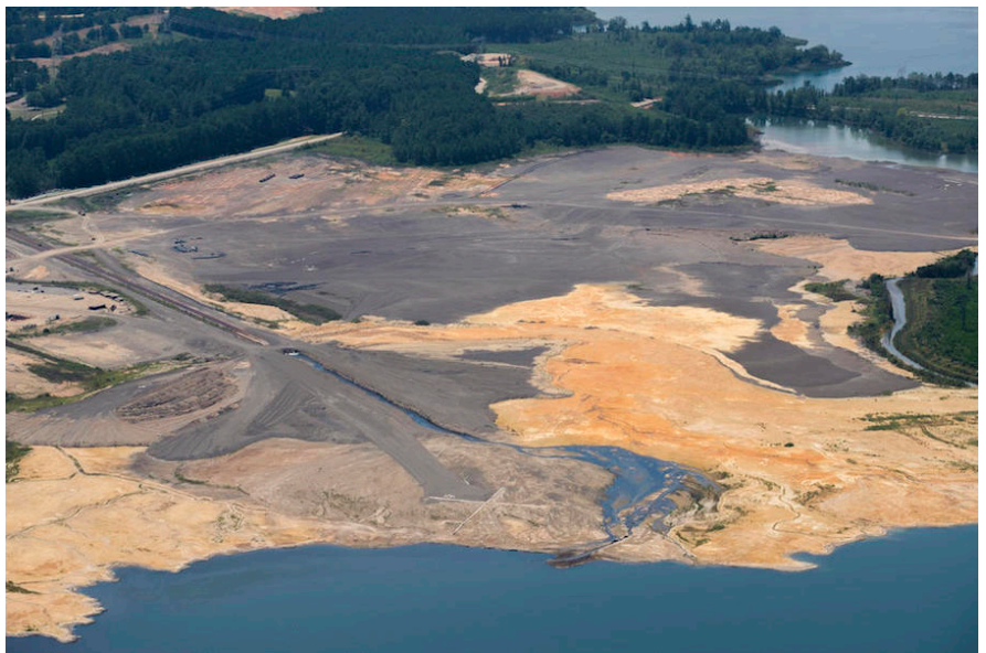
Georgia Power's Plant Scherer (article on next page).
