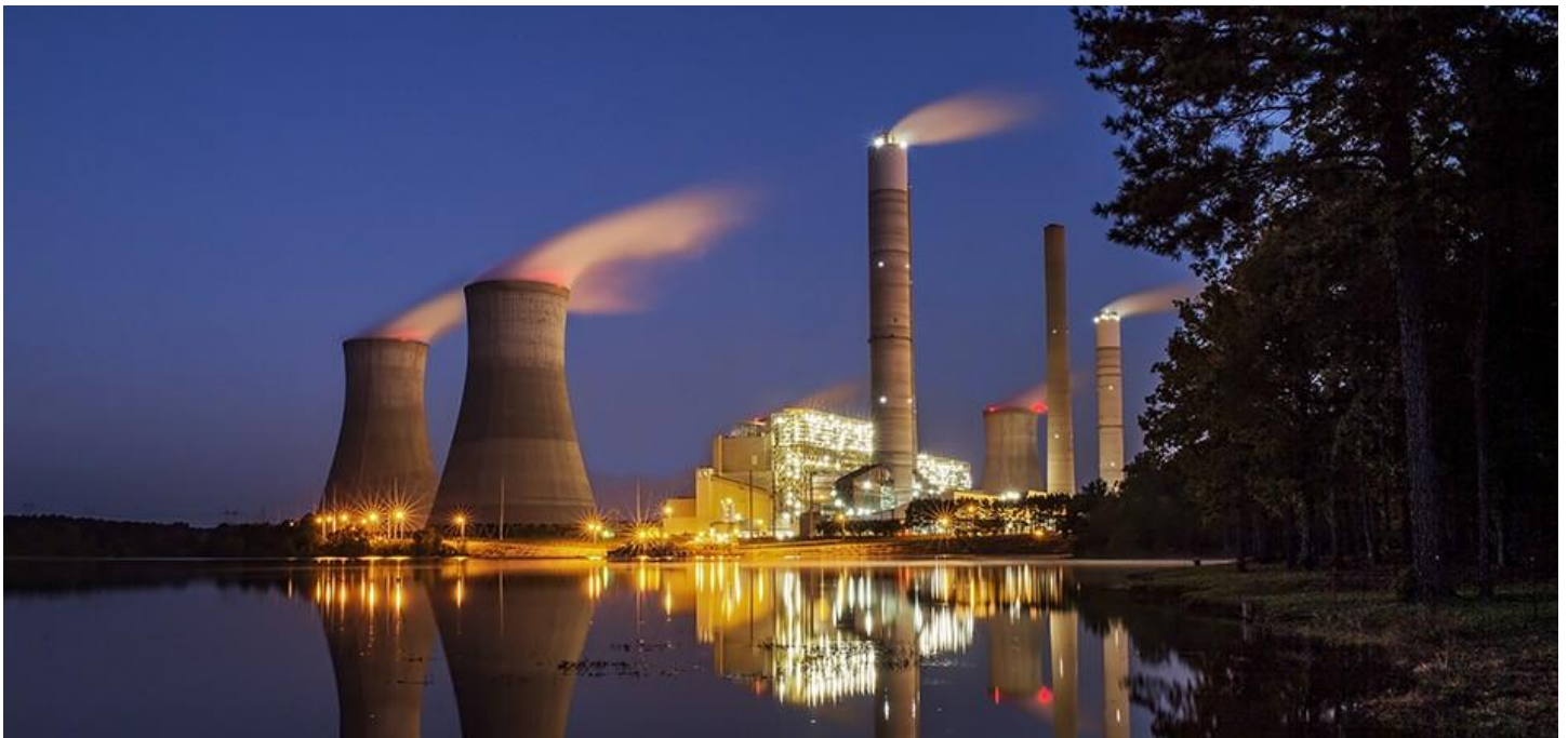
Georgia Power's Plant Scherer in Monroe County, GA.
