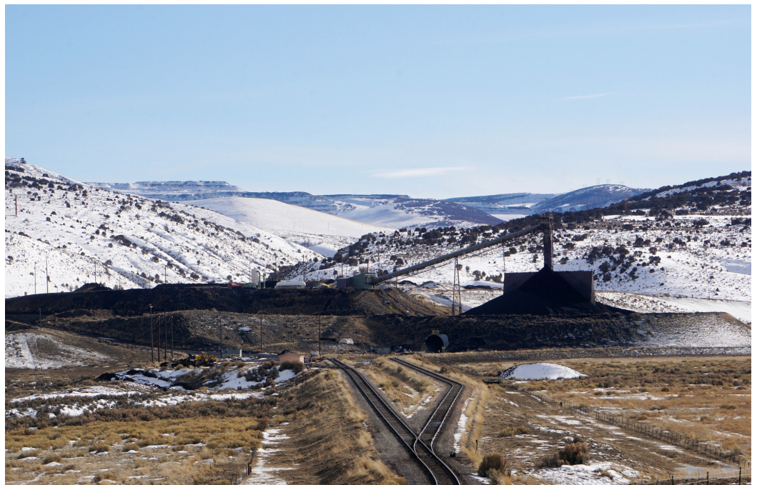
Colowyo Coal Company which supplies coal to Craig Station in Moffat Co, CO.
