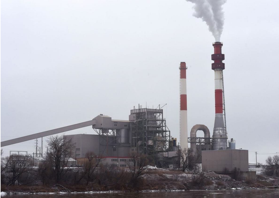
Lewis and Clark Generating Station in Montana.
