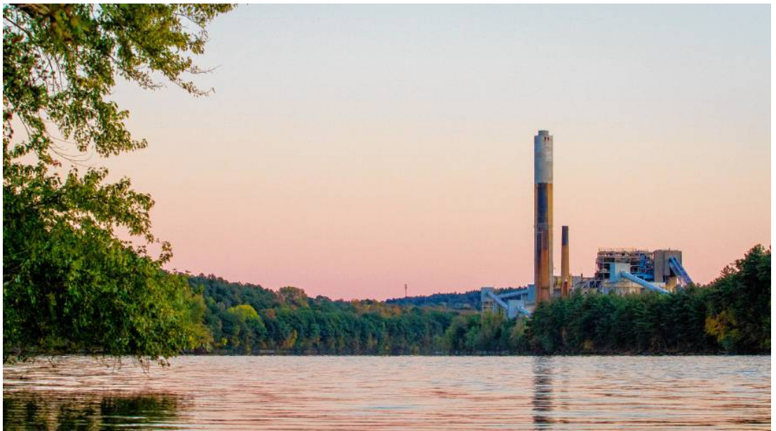
Merrimack Station in Bow, New Hampshire.
