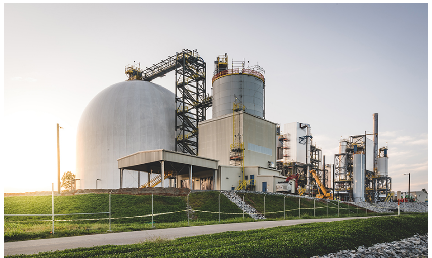
Buck Steam Station Plant in Rowan County, NC.
