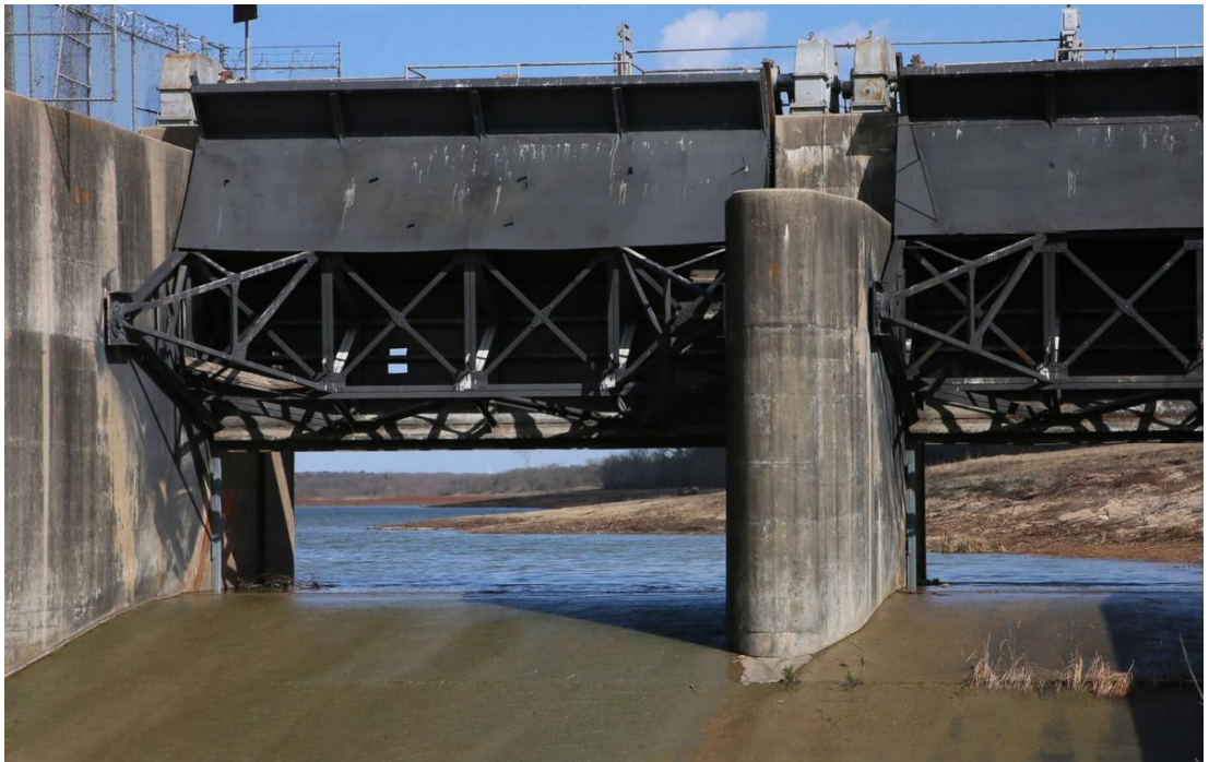
View of the Lake Creek Power Plant near Riesel, TX.
