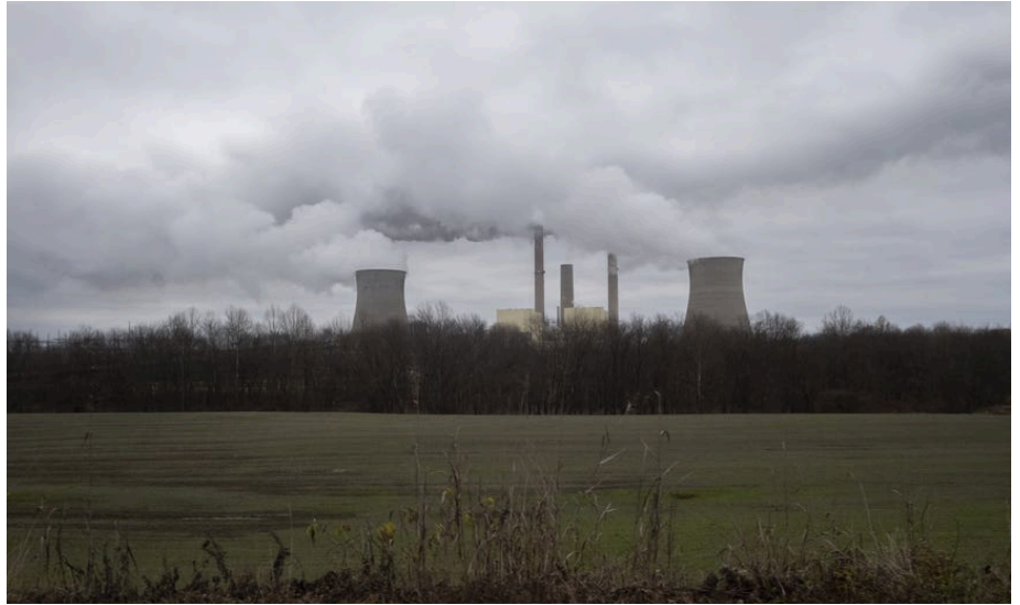
Gen. James M. Gavin Power Plant in Cheshire, OH.
