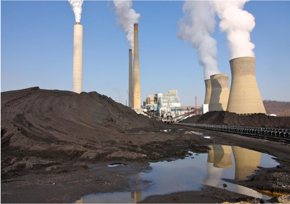
John E Amos Power Plant in Winfield, WV
