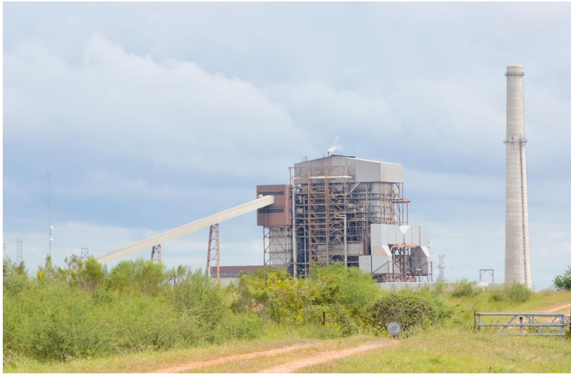
Coletto Creek Power Plant in Goliad County, TX
