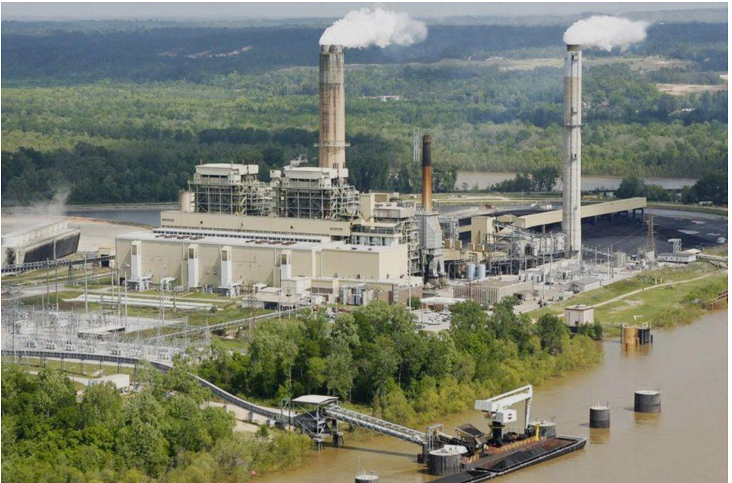
Lowman Power Plant, Jackson, Alabama
