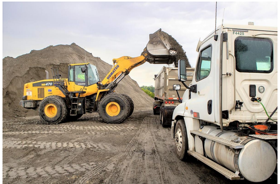
Removing fly ash from the Santee Cooper Site (2017)
