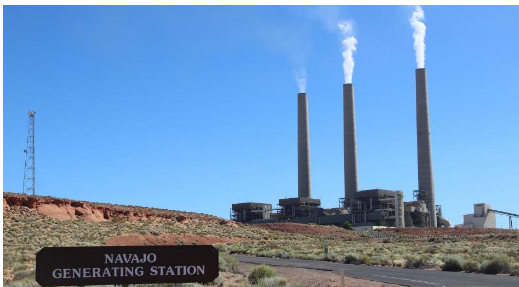
Navajo Generating Station
