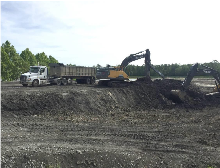
Excavating Coal Ash from Ponds at Grainger Generating Station
