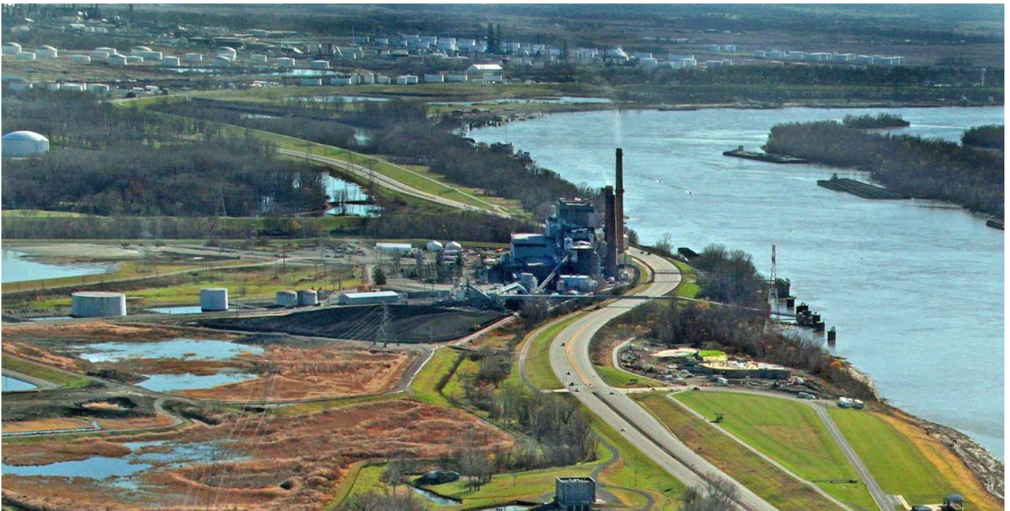
Wood River Power Plant
