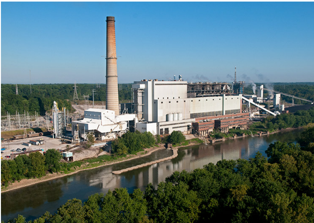
Wabash River Generating Station
