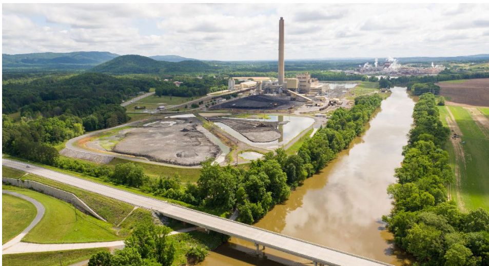
Georgia Powers Plant Hammond
