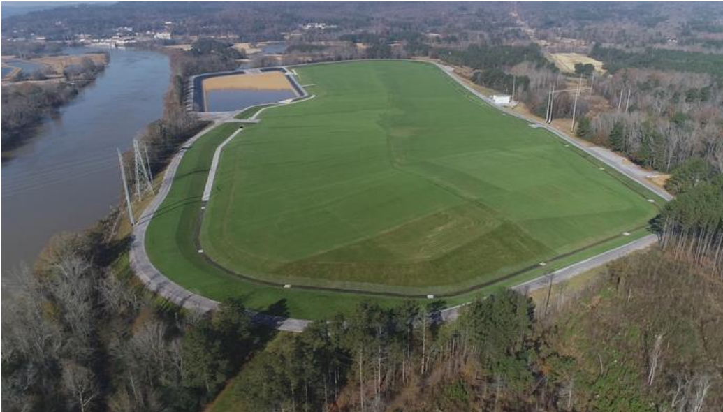
Alabama Power's Plant Gadsden
