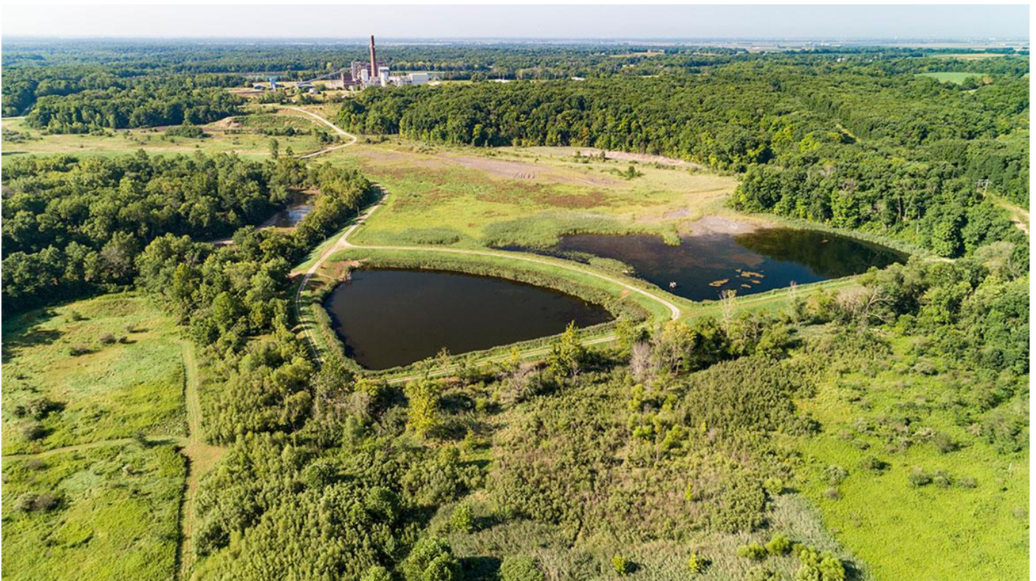
Coal Ash Ponds at Vermilion Power Station
