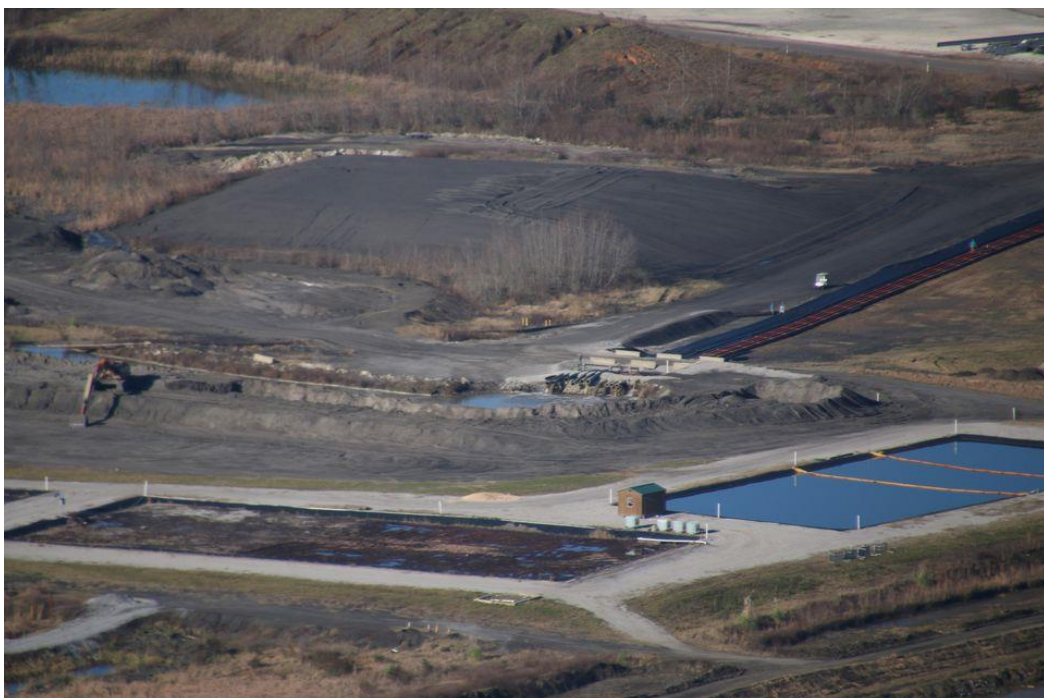
Coal Ash Pond at Alabama Power's Plan Barry
