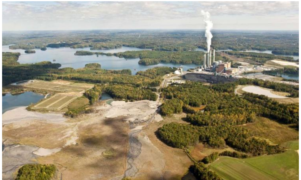
Belews Creek Steam Station
