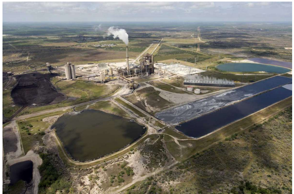
San Miguel Power Plant
