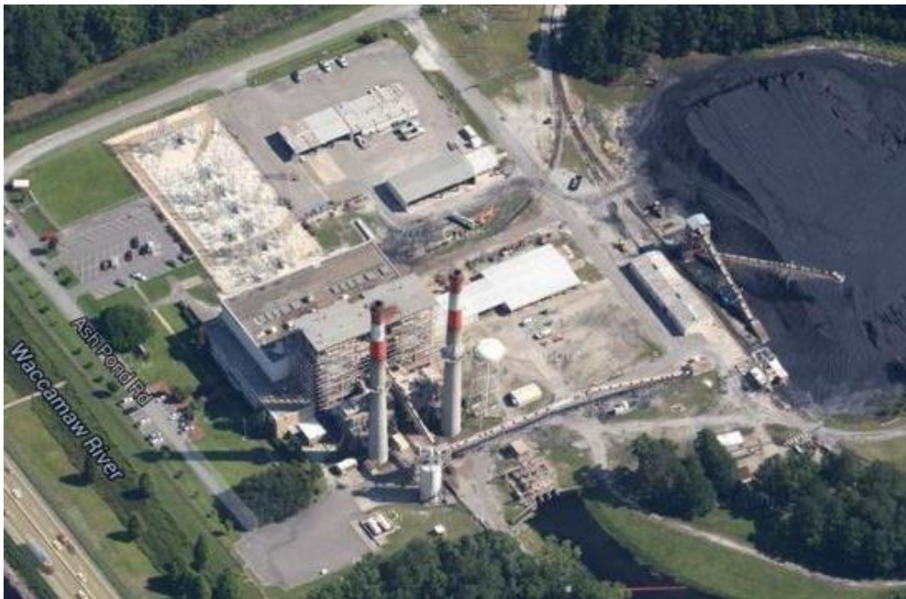
Grainger Generating Station
