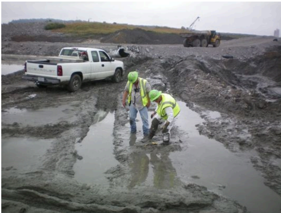
Unprotected workers in wet coal ash sludge during the cleanup of the spill at the TVA's Kingston Fossil Plant
